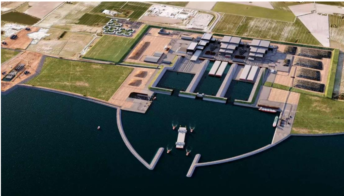
Figure 1: Tunnel Harbour Rødbyhavn
